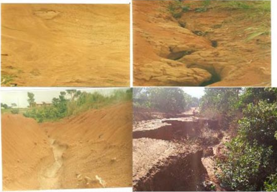
Fig 3: Soil Erosion (consequences of excess rainfall) (Source: Authors field work, 2010)
