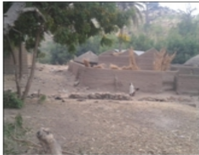
Fig. 3: Good Traditional House
