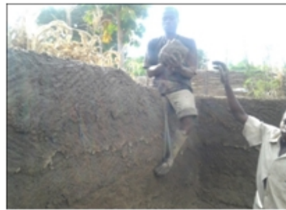
Fig. 4: Construction of Wall
