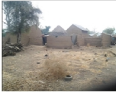
Fig. 1: Dilapidated Traditional House
