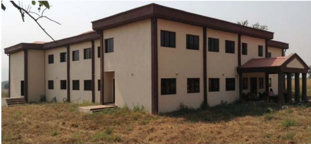
Project 1: The NERDC new library complex at Sheda, Abuja. Source: Authors' Fieldwork, 2015
