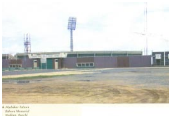
Fig. 5: Abubakar Tafawa Balewa Memorial Stadium.
