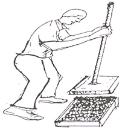
Figure 1: Manual ramming method used in Shelf Production Source: Studio Practice
